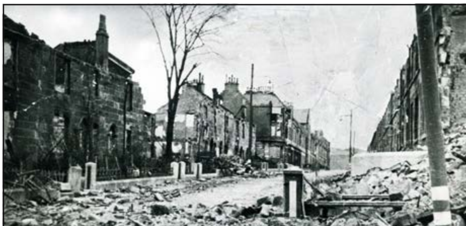
Clydebank blitz damage
